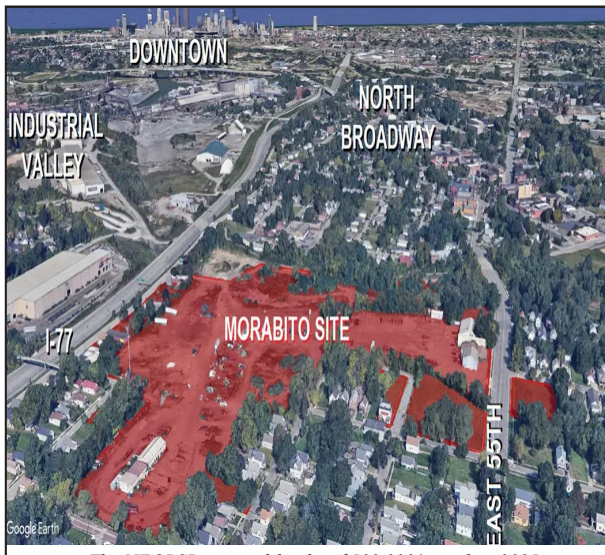
The NEORSD acquired land at $500,000/parcel in 2025 to support the Morabito Site development of a hyperscale data center
